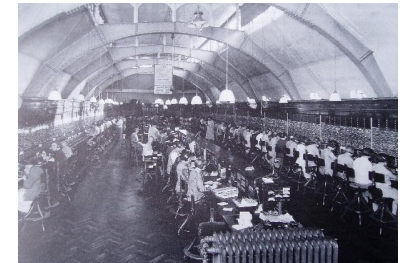
Telephone Central Office in London, 1926
