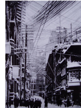
New York Telephone Cabling, 1888
